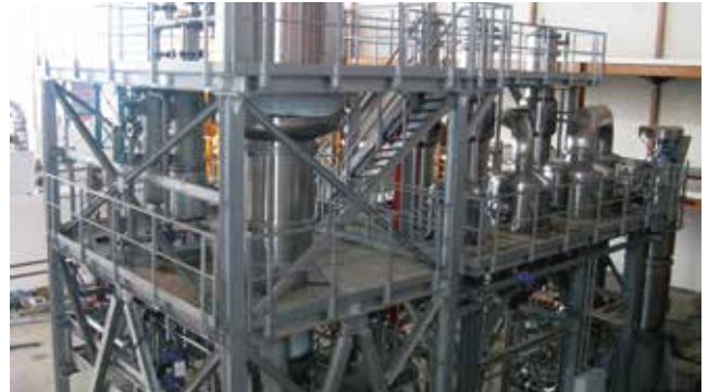
● COMPLETE INSTANT COFFEE PLANT INDONESIA, 2008
